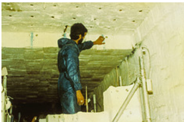
Figure 8.4 Re-lining a furnace with refractory ceramic fibre blocks
