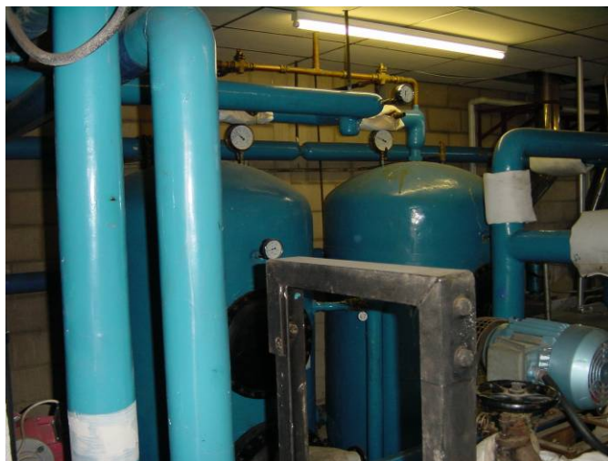
Figure 8.2 Insulation (lagging) to pipework and calorifiers
