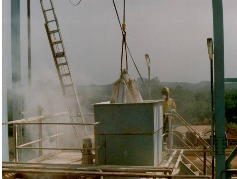
Photograph 2 – Adding Hydrated Lime
