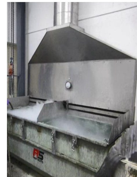
Local Exhaust Ventilation (LEV)
