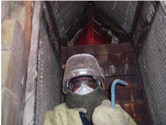
Photograph 3 – Refractory Worker Wearing His Typical PPE
