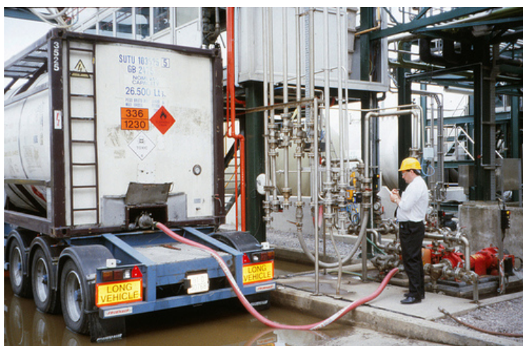
Figure 9.3 – Delivery of methanol from tanker
