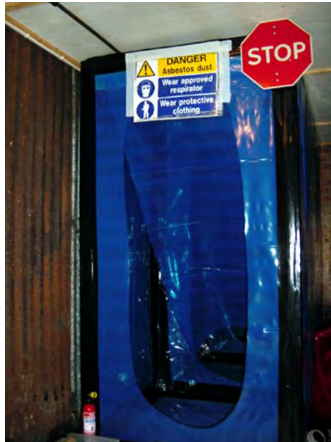
Figure 6.4 – Enclosure (airlock entry)
