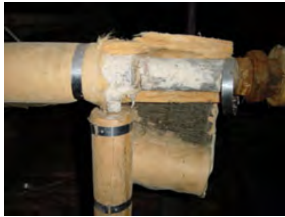
Figure 5.16 – Asbestos residues beneath mineral fibre insulation
