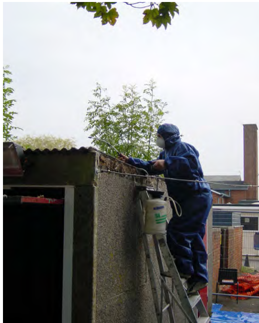
Figure 6.10 – Wetting of asbestos cement
