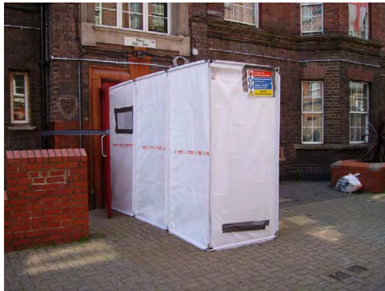
Figure 6.5 – Enclosure (temporary airlock system)
