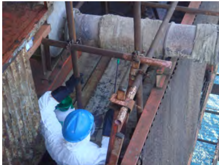
Figure 6.9 – Wetting of asbestos textile insulation
