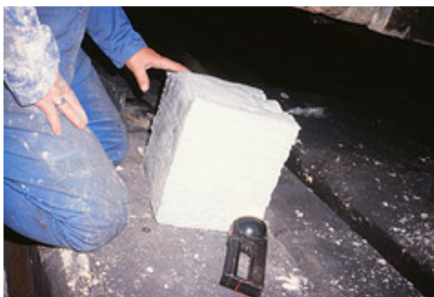
Figure 8.5 Re-lining a furnace with refractory ceramic fibre blocks
