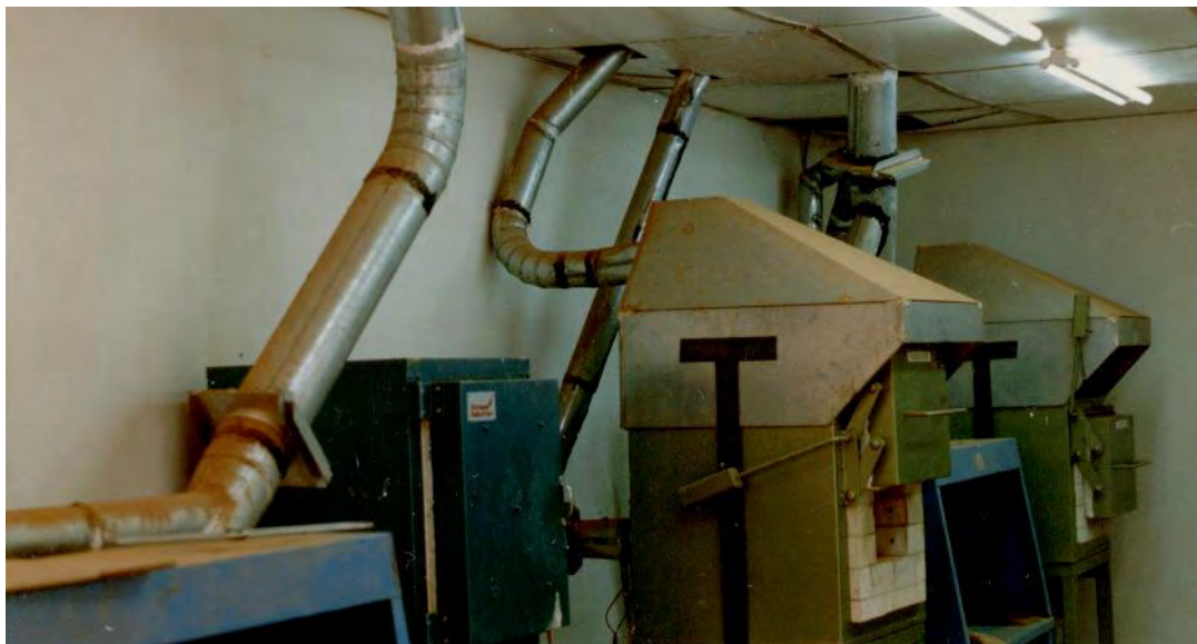
Figure 10.3 – Laboratory Ventilation System Ducts
