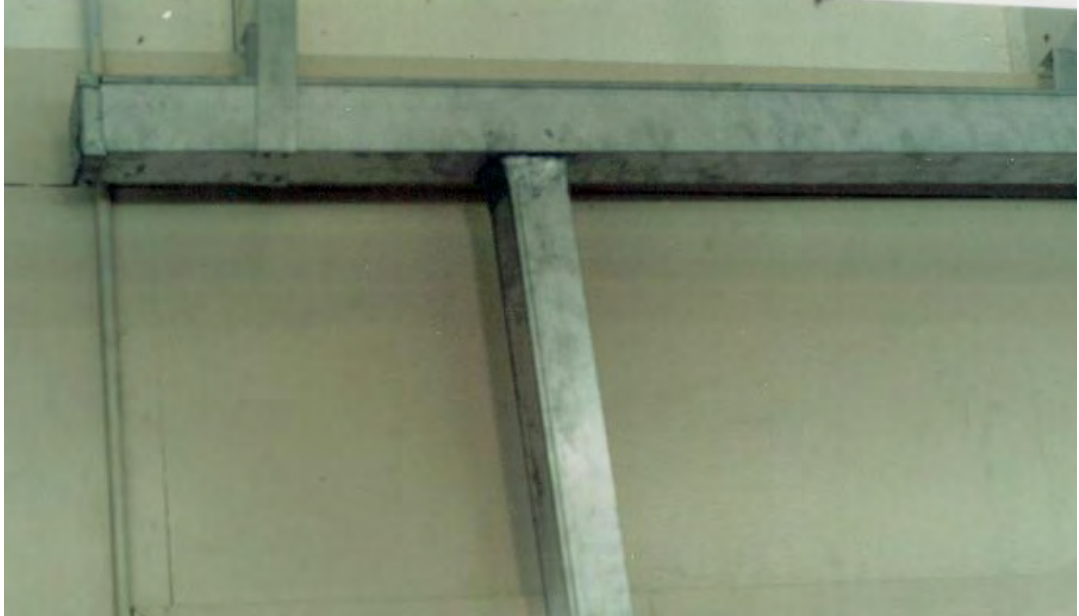
Figure 10.5 – Close-up of “T” Joint in Ductwork
