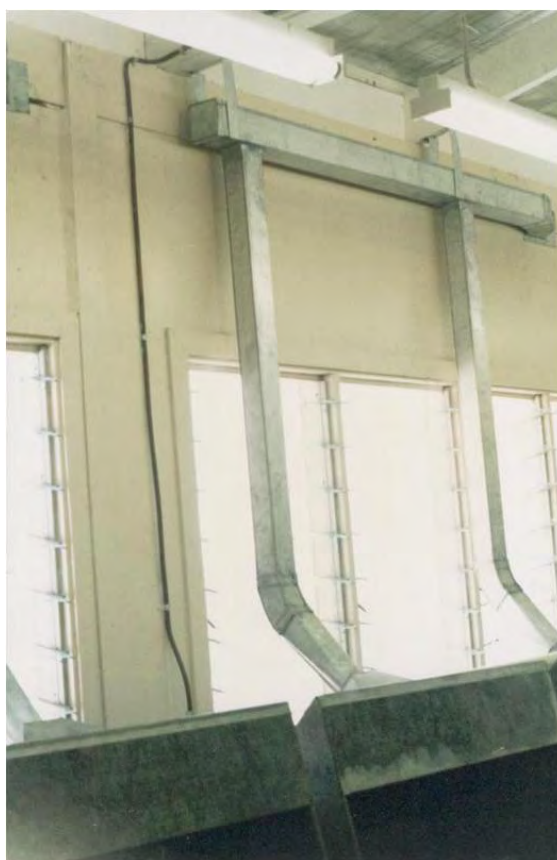
Figure 10.4 – Ductwork for Extraction System
