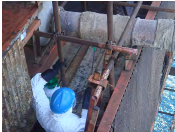
Figure 6.9 – Wetting of asbestos textile insulation
