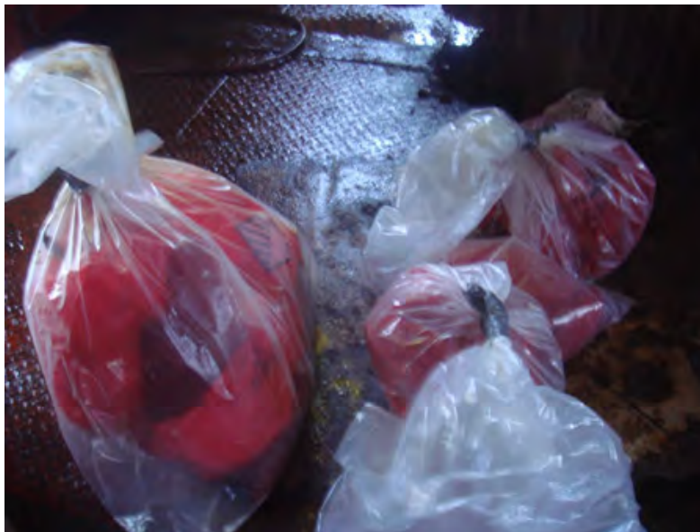
Figure 6.12 – Asbestos waste bags (double bagged)
