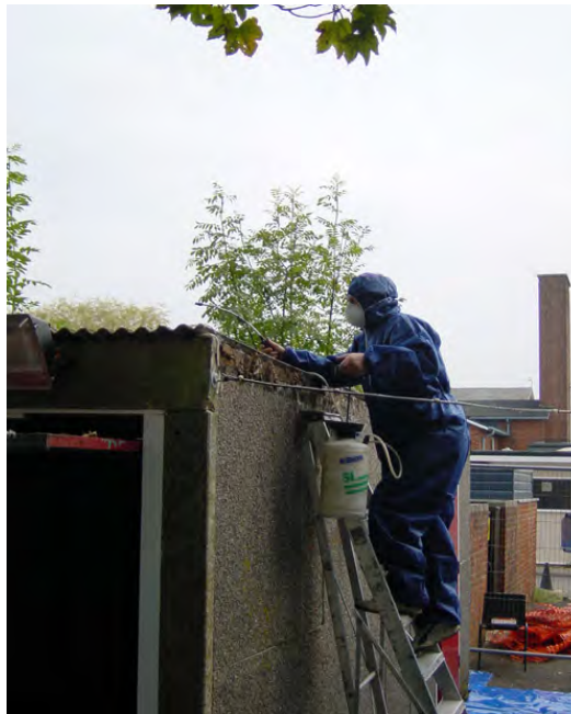
Figure 6.10 – Wetting of asbestos cement
