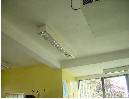
Figure 5.10 Asbestos based textured decorative coating to ceiling
