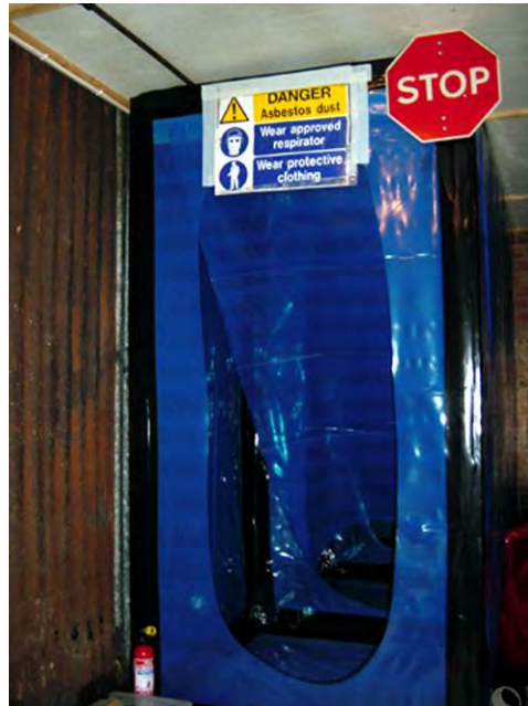
Figure 6.4 – Enclosure (airlock entry)
