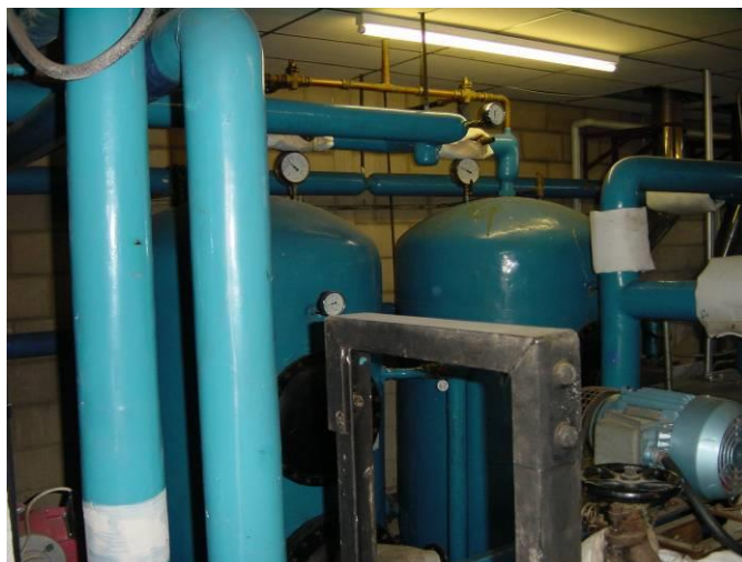
Figure 8.2 Insulation (lagging) to pipework and calorifiers
