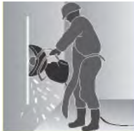
Figure 5.6 – Use of concrete saw requires application of high force and sustained awkward postures of back and neck
