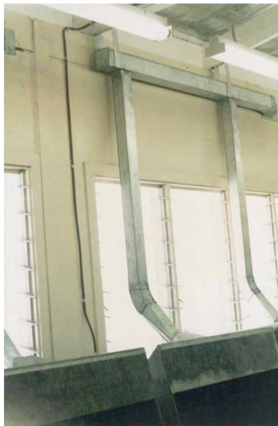
Figure 10.4 – Ductwork for Extraction System
