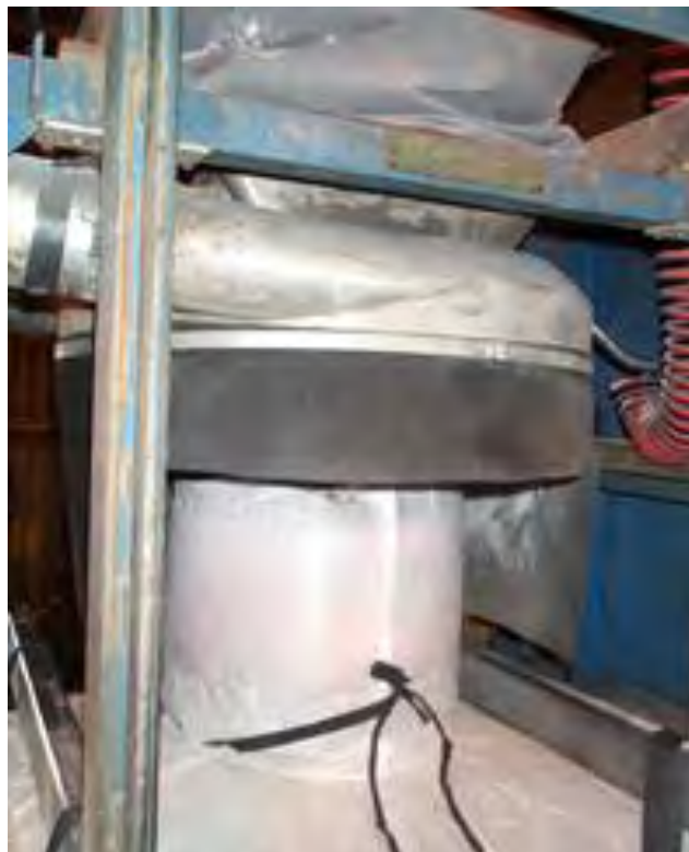
Figure 10.11 – Local Exhaust Ventilation During Bag Filling
