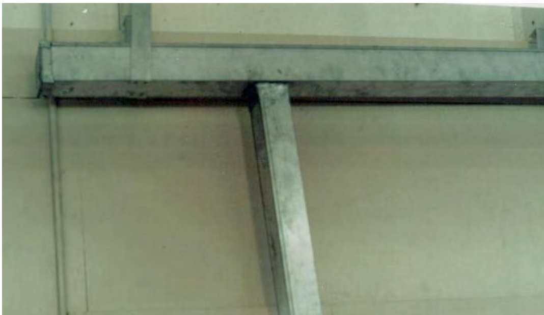
Figure 10.5 – Close-up of “T” Joint in Ductwork
