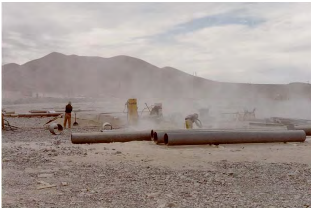
Figure 10.2 – Sand Blasting Steel Pipes
