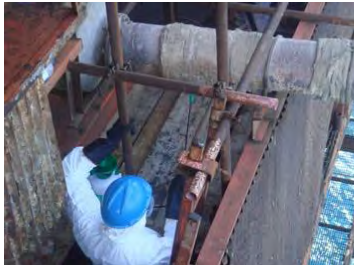
Figure 6.9 – Wetting of asbestos textile insulation
