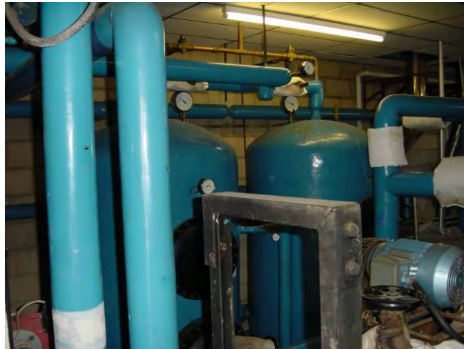
Figure 5.2 Insulation (lagging) to pipework and calorifiers
