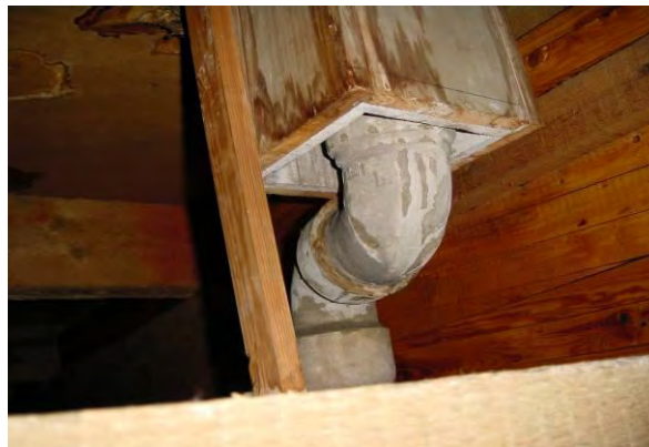
Figure 5.6 Asbestos insulating board lining panels and asbestos cement flue pipe
