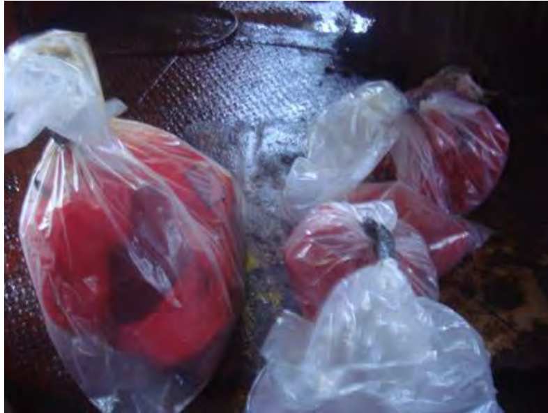
Figure 6.12 – Asbestos waste bags (double bagged)
