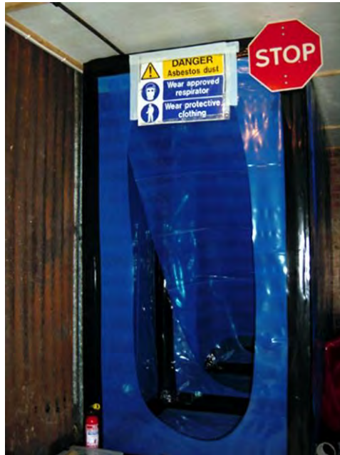
Figure 6.4 – Enclosure (airlock entry)
