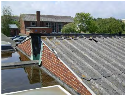
Figure 5.8 Asbestos cement corrugated roof panels
