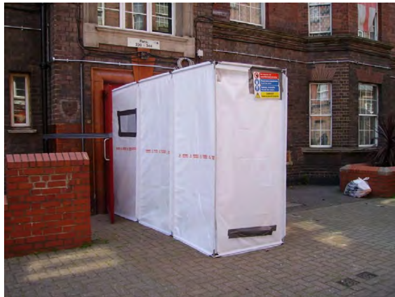
Figure 6.5 – Enclosure (temporary airlock system)
