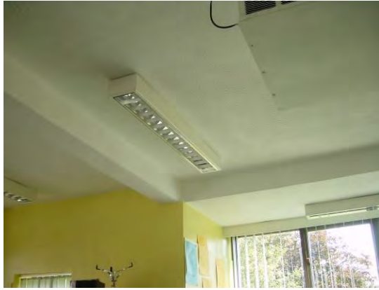
Figure 5.10 Asbestos based textured decorative coating to ceiling
