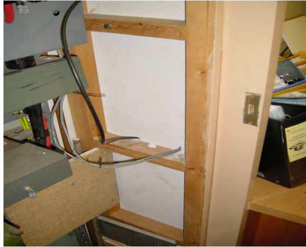
Figure 5.4 Asbestos insulating board internal wall panels
