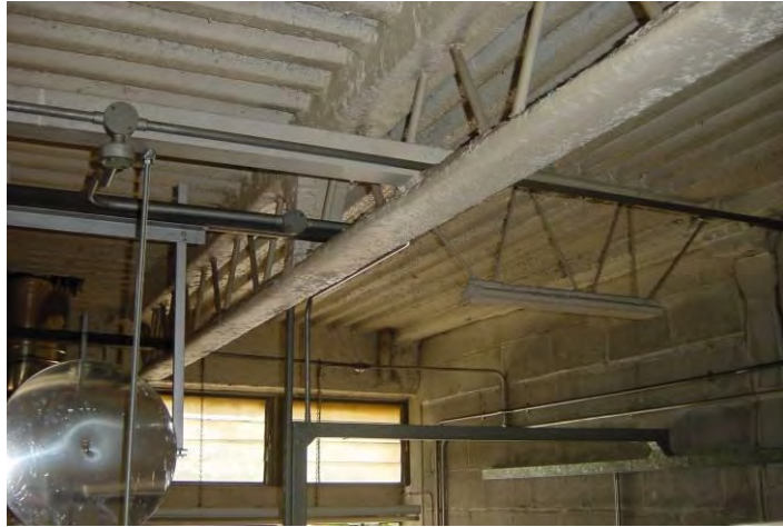
Figure 5.1 Spray coating to support girders and ceiling
