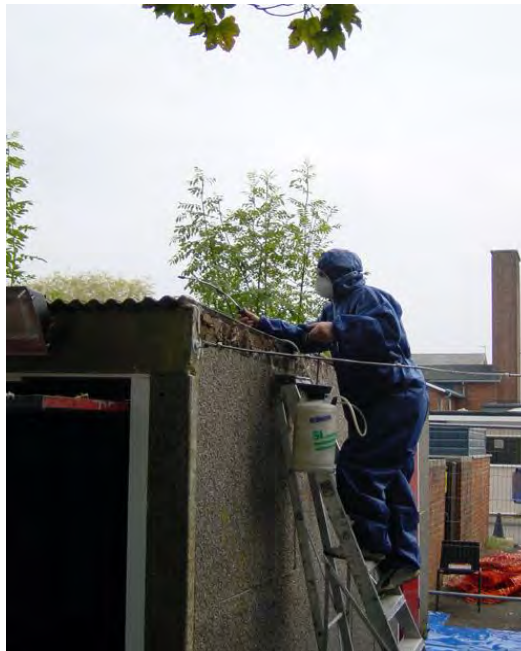
Figure 6.10 – Wetting of asbestos cement
