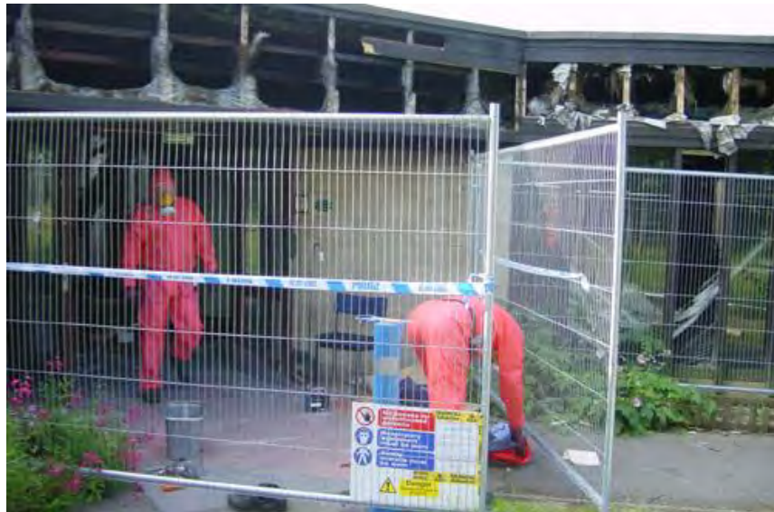
Figure 4.2 Disposable coveralls and full-face respiratory protection
