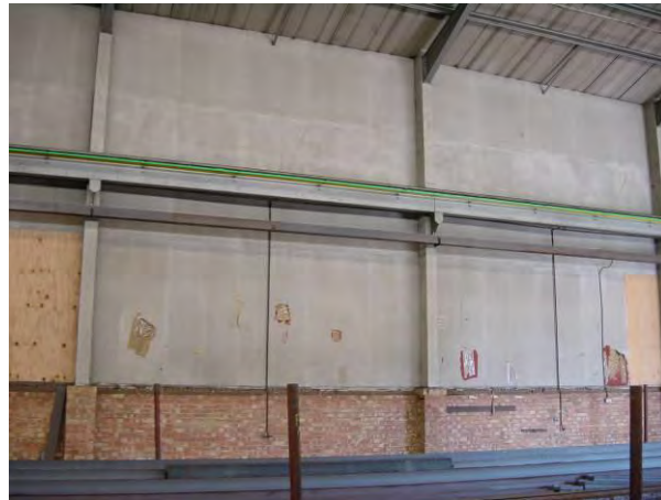
Figure 5.5 Asbestos insulating board wall lining panels
