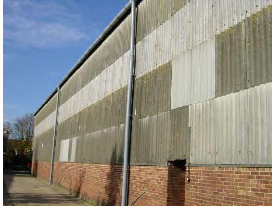
Figure 5.7 Asbestos cement external wall panels
