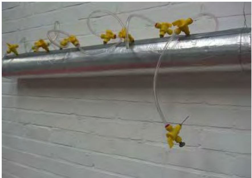
Figure 6.8 – Wet injection equipment (last needle removed for clarity)
