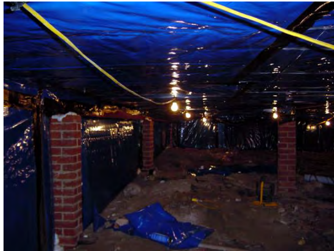
Figure 6.3 – Enclosure (service duct under floor)
