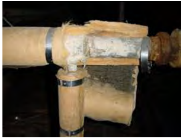
Figure 5.16 – Asbestos residues beneath mineral fibre insulation
