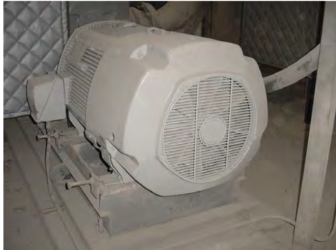
Figure 4.1 - Totally-enclosed fan cooled electric motor
