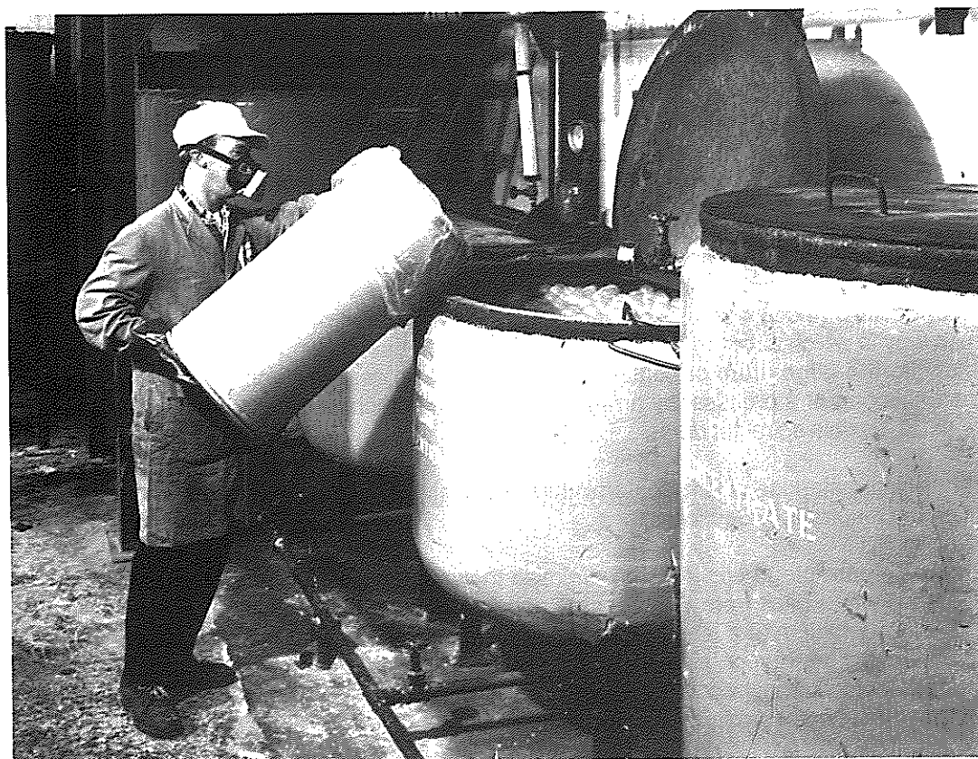
Figure 5.1 Plastic balls reduce evaporation from liquid surface (photograph courtesy of Capricorn Chemicals Ltd, Stratford, London).
