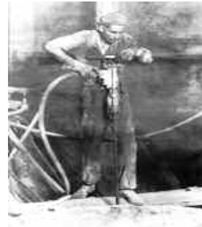
Lewis Hine, 1931, pneumatic drill
